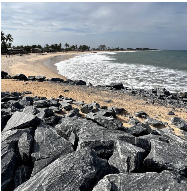
Sea-level rise challenging traditional coastal defence structures at Ghana's eastern coast.
