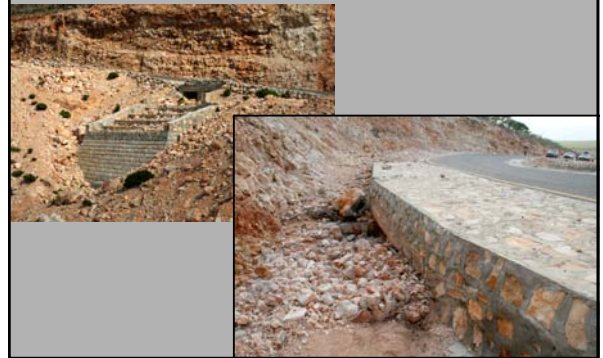
Example of improper culvert dimensions causing blockage resulting in erosion of roads
